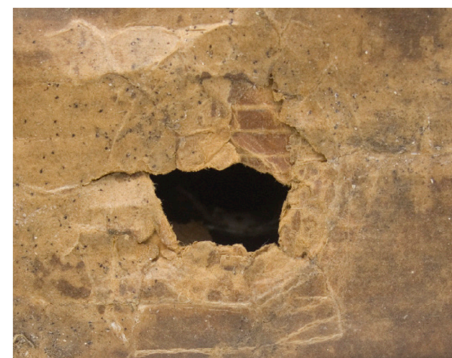
Figure 8: The repaired hole. The inserted rods are completely hidden from view by the overlying layers of consolidated paper. Photo: Christine Frohnert, 2010.
