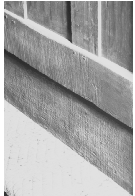
Figure 1. Pit saw marks vs hand saw marks. Courtesy of John Childs
