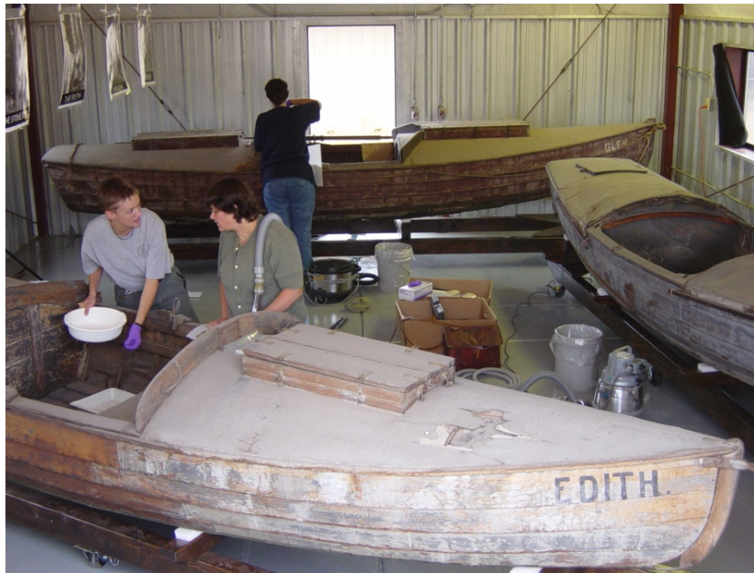
Fig. 5. Dry cleaning the wooden boats (Photograph by M. Quinn)
