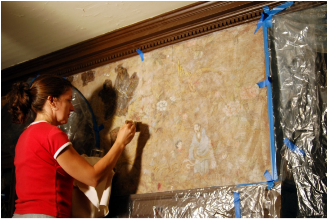
Fig. 4. Applying melted cyclododecane by brush (Photograph by Judith Bohan)
