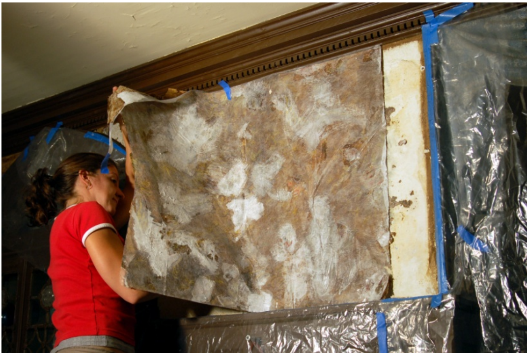
Fig. 5. Removal of the wallpaper with facing using a Teflon spatula (Photograph by Judith Bohan)
