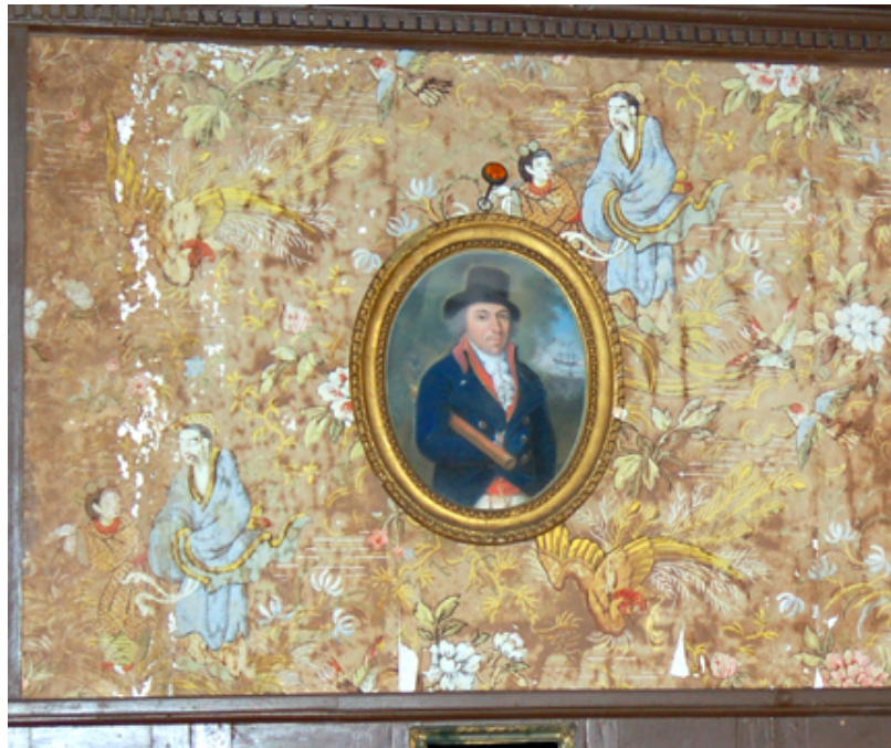
Fig. 3. The Chinoiserie wallpaper showing losses and dark stains (Photograph by Michaela Neiro)
