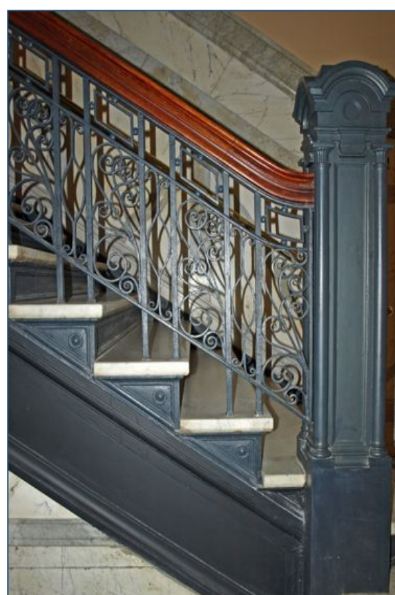
West Staircase, cast and wrought iron
