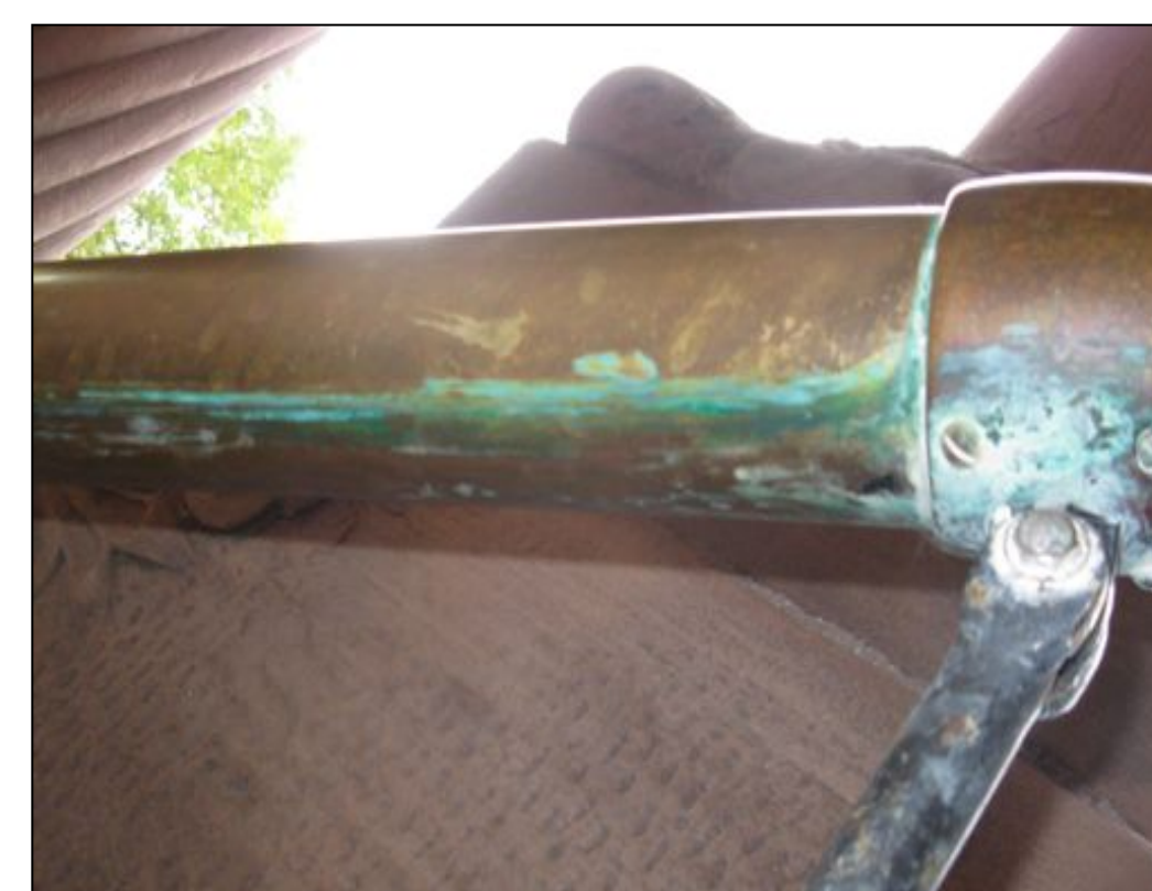
Brass handrail, Met-All polish residue
