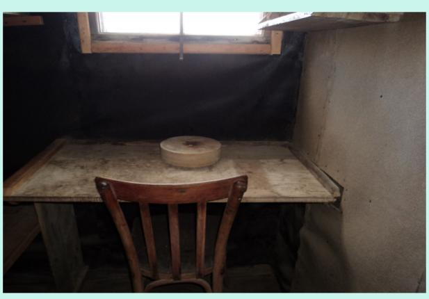
The hut was made by a Norwegian factory ("Jowengstrom"), which manufactured this type of construction in early 1900. It was transported disassembled and was assembled in site. The original building materials are wood, metal (nails and anchors) and glasses (windows). The expedition also used tar paper, linoleum, and textiles as barriers for the cold climate.
