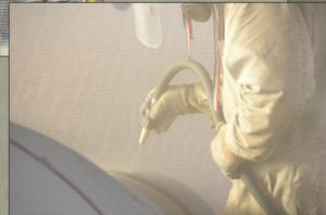
**Coating System:** NPS requirements were for a long-term stable primer and paint system that would withstand the harsh environment for a minimum of five years. In consultation with Keith Lucas, director of the Center for Corrosion Science and Engineering at the Naval Research Laboratory, Amercoat 68HS was selected. This zinc-rich, epoxy-based primer is designed for outstanding resistance in a marine environment.
