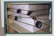
Fragile boxed objects held on shelves with Seismic Shock Cord Restraints.
