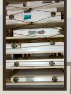
Close up—aluminum grommet used to attach Seismic Shock Cord Restraint to existing library shelving provides easy release for access.
