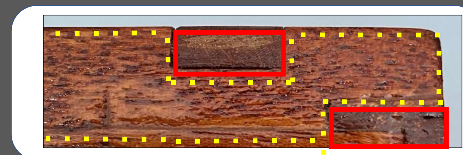
Figure 5. Side profile of deckle joint.
