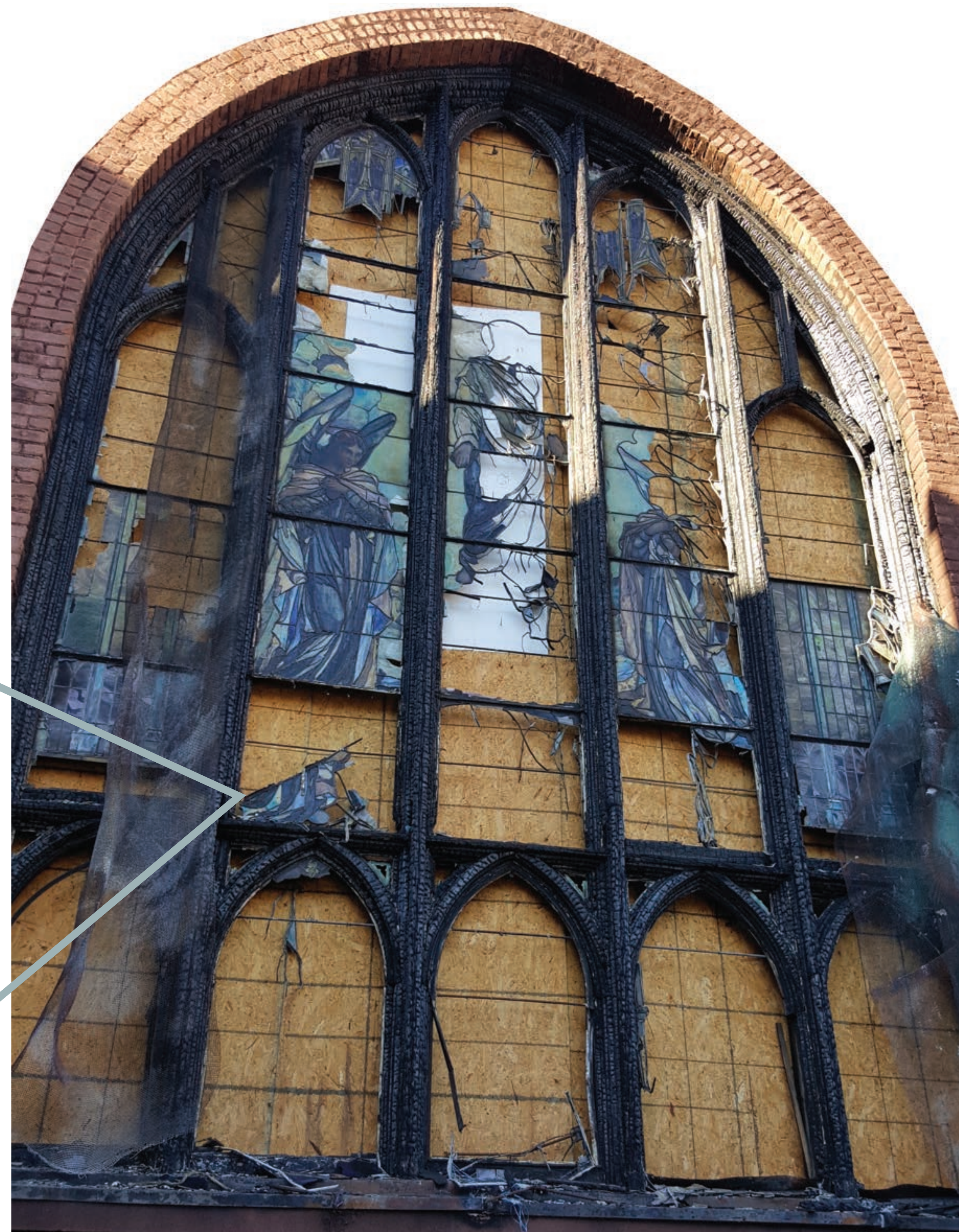
"Ascension Window", J & R Lamb Studio ca. 1912. Brooklyn, NY. ext. following a structure fire in 2016. Image courtesy of Bovard Studio, Inc.
