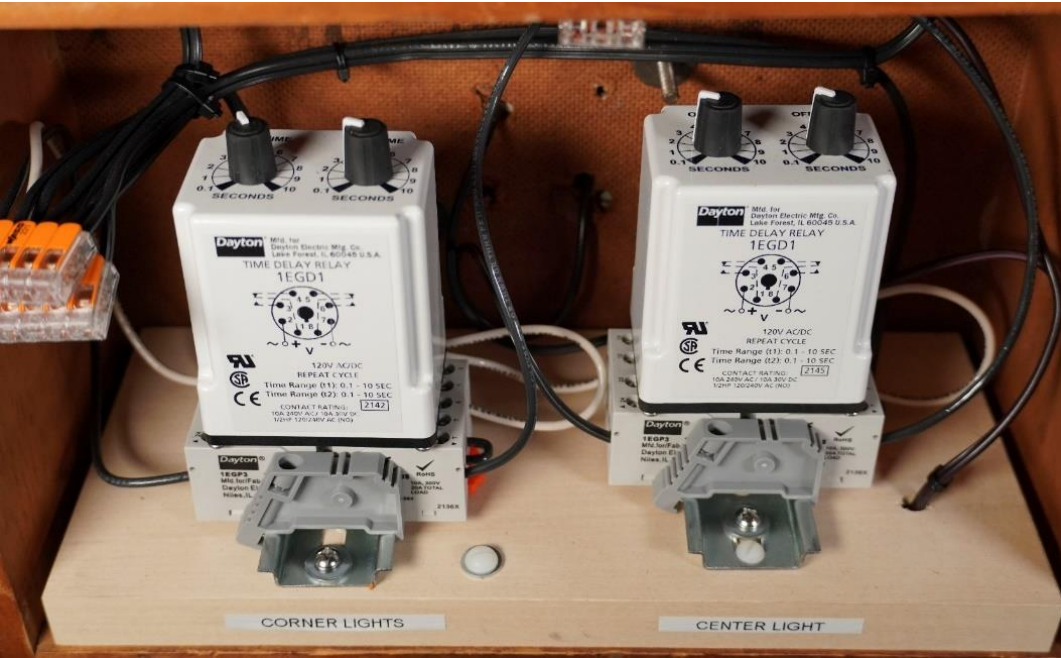
FIGURE 6 Detail of new relays and wiring.
