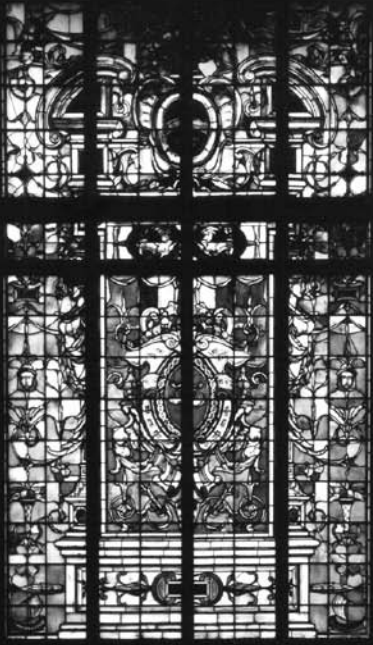
Indianapolis Federal Courthouse Stained Glass Conservation
