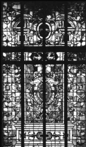
Indianapolis Federal Courthouse Stained Glass Conservation
