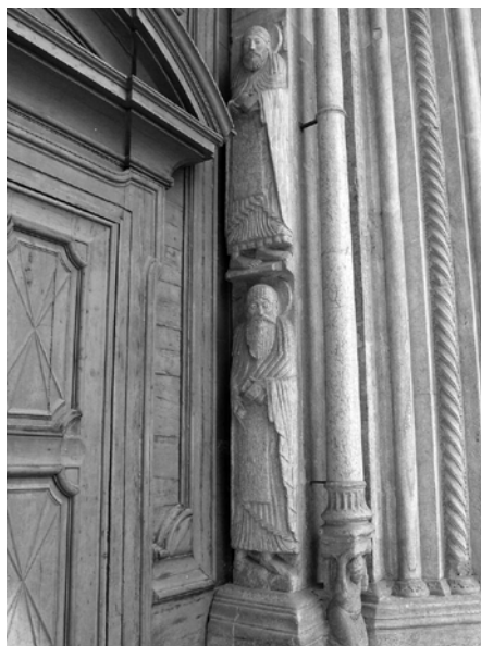
Figure 3. Treated prophets 15 years later. The top statue is cleaned using chemical and bead blasting techniques while the bottom is cleaned using a long pulsed Nd:YAG laser.
