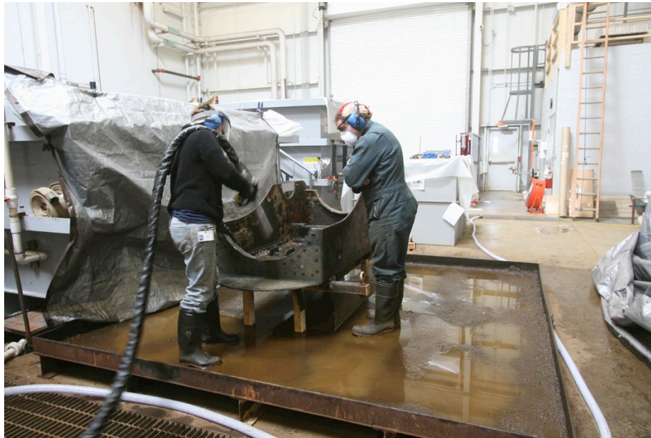
Figure 4 (above). Mariners' staff member Laurie King is seen wearing all of the appropriate PPE for dry ice blasting treatment: ear protection, eye protection, respirator mask, cold protection gloves, long sleeves, trousers, and boots. Image courtesy of The Mariners' Museum and Park.
