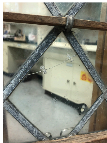
Figure 9. Detail of B-72 staples stabilizing a broken pane. Courtesy of the Colonial Williamsburg Foundation.
