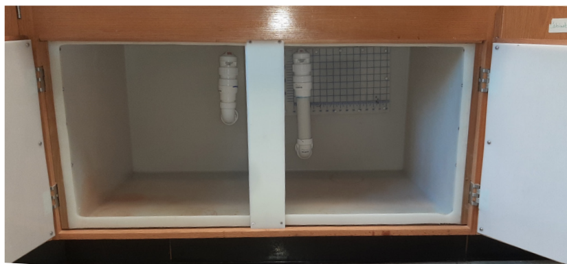
Figure 5. Empty acid cabinet with partition for two separate compartments, lined with HDPE and LDPE sheets, the back access panel of reused cutting board.
