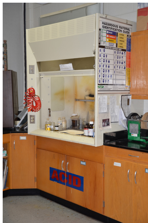
Figure 4. Overall view of direct vented fume hood above acid cabinet.
