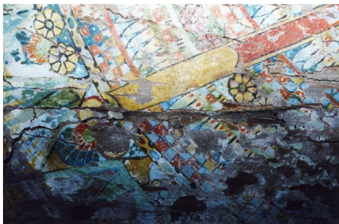
Figure 6. Detail of flaking polychrome paints in the area of the partially lacquered collar.
