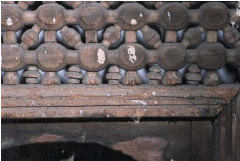
Figure 3. Detail of damage to mashrabiyya No. 2979 in the Museum of Islamic Art in Cairo.
