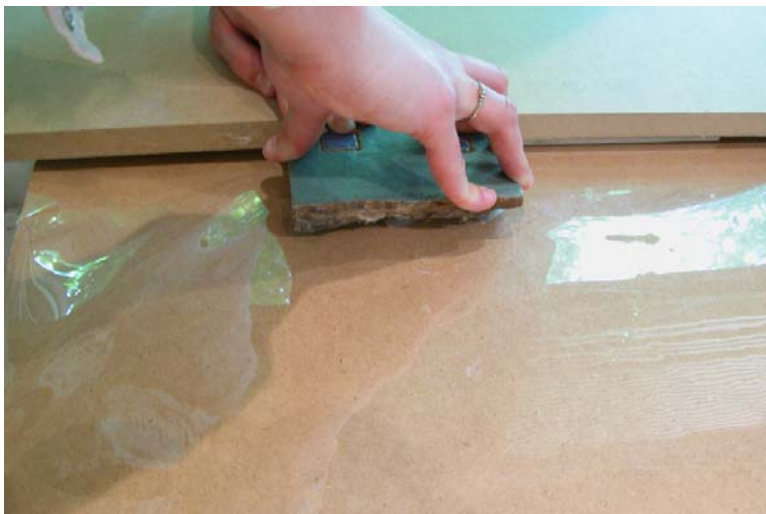
Figure 7. Compressing a tile.
