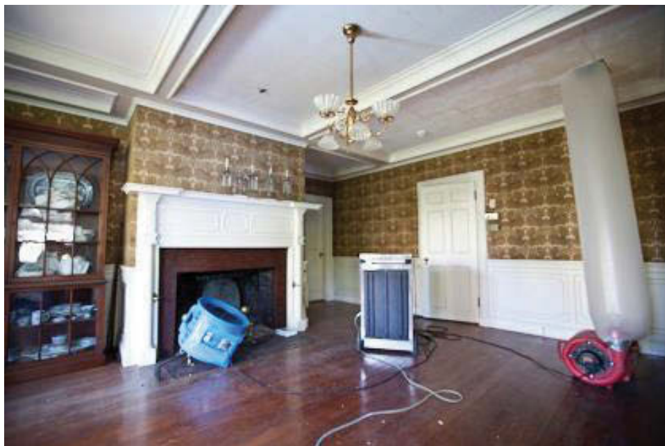
Fig. 9. Dehumidifiers and blowers in place to reduce humidity (Courtesy of Kathy Tarantola)
