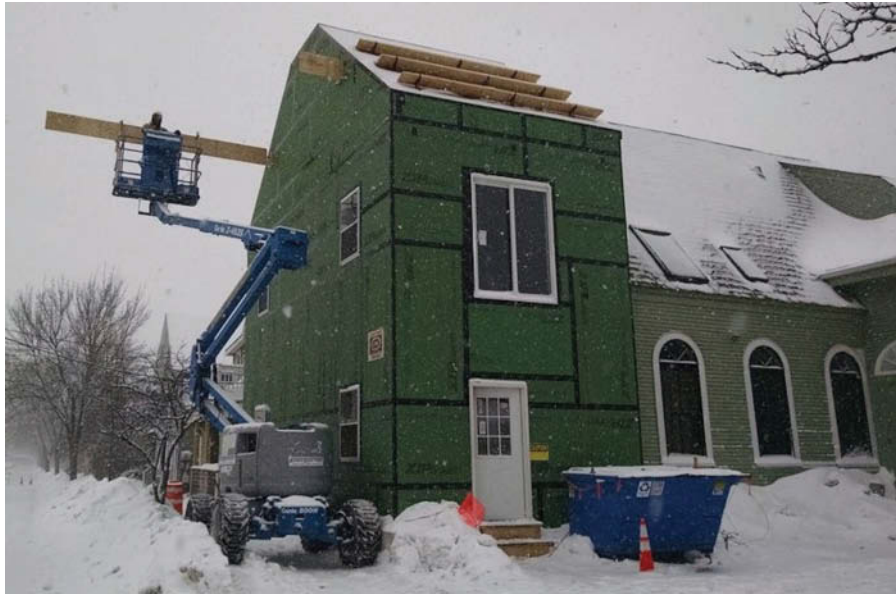
Fig. 9. Protective structure enclosing the apse (Courtesy of Lost Shul Mural Project and Bob Neeld, PE)
