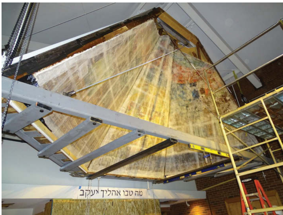
Fig. 19. Mural lifted to viewing height and steel floor support being removed (Courtesy of Bob Neeld, PE)
