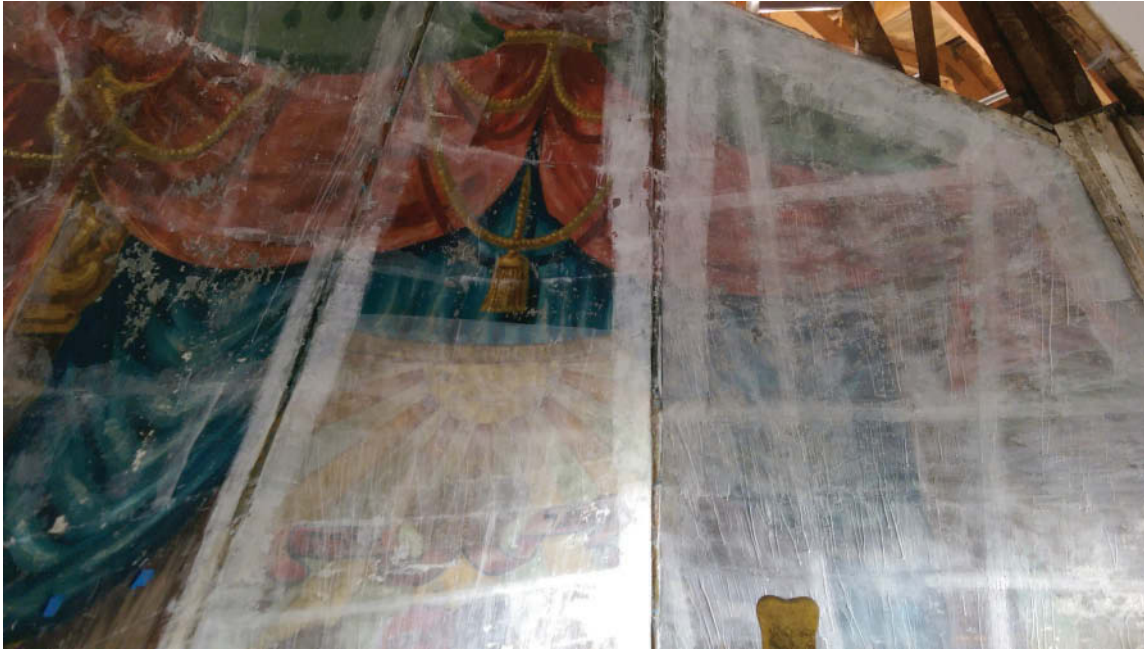
Fig. 11. The left side of the mural is faced with Crepeline. The right side has cyclododecane applied over fiberglass Micro-mesh on top of the Crepeline facing (Courtesy of Bob Neeld, PE)
