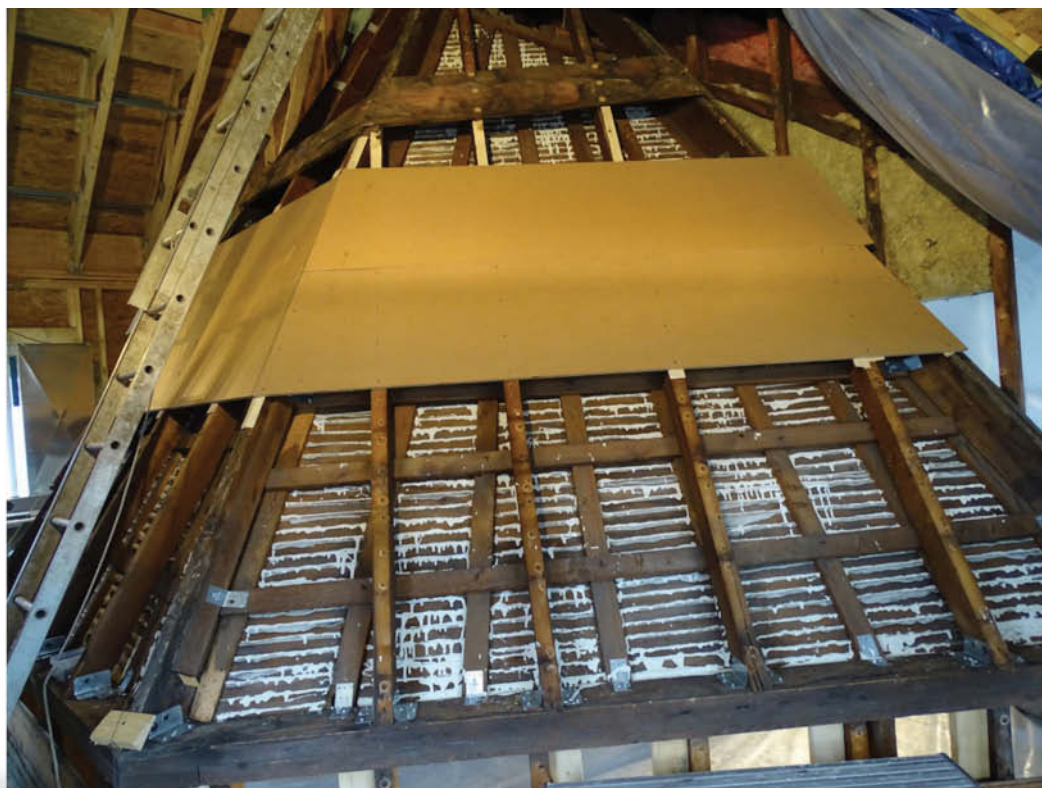
Fig. 10. Reverse of the mural showing plaster keys from the back and the newly created key extensions, metal reinforcing brackets, and new plywood roof sheathing (Courtesy of Bob Neeld, PE)
