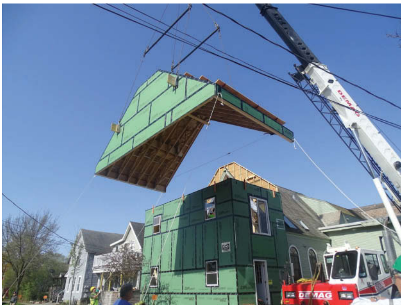
Fig. 16. Crane removing roof (Courtesy of Lost Shul Mural Project)
