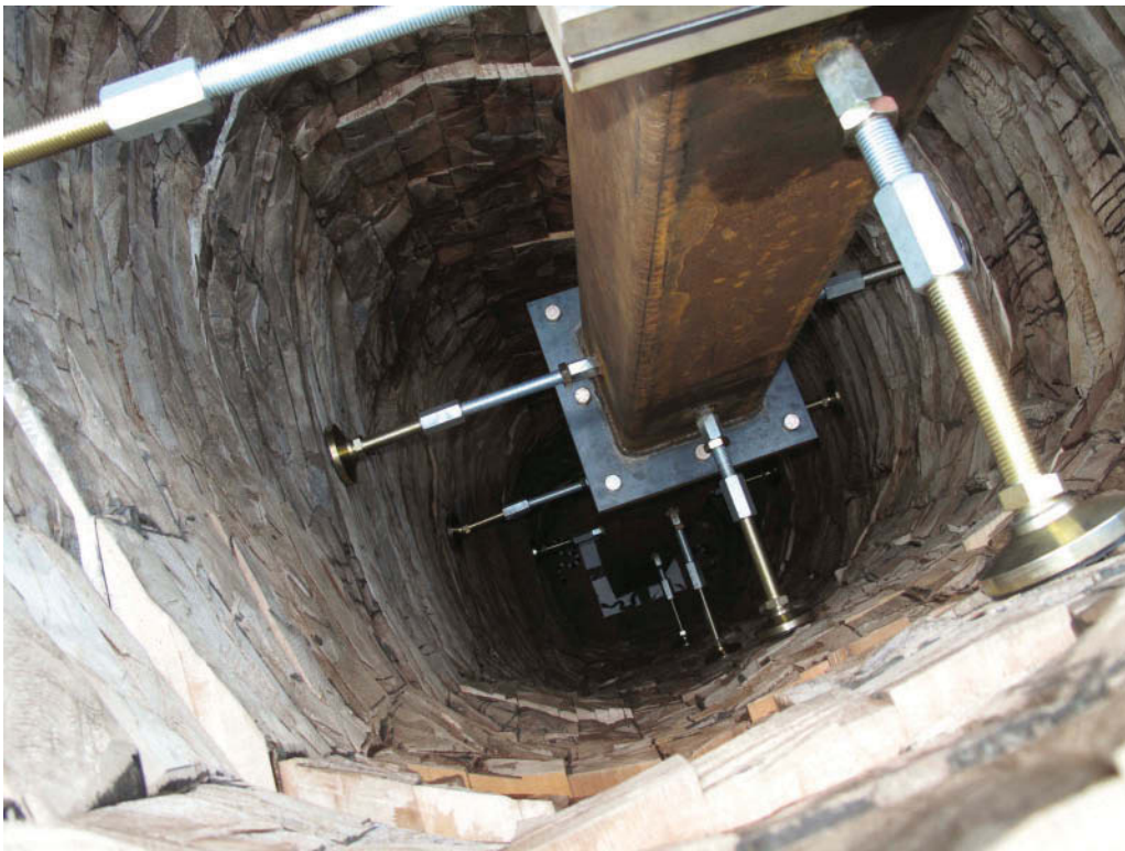
Fig. 12. The pressure-fit posts as installed (Courtesy of Ursula von Rydingsvard, photograph by AJ Bucknall)
