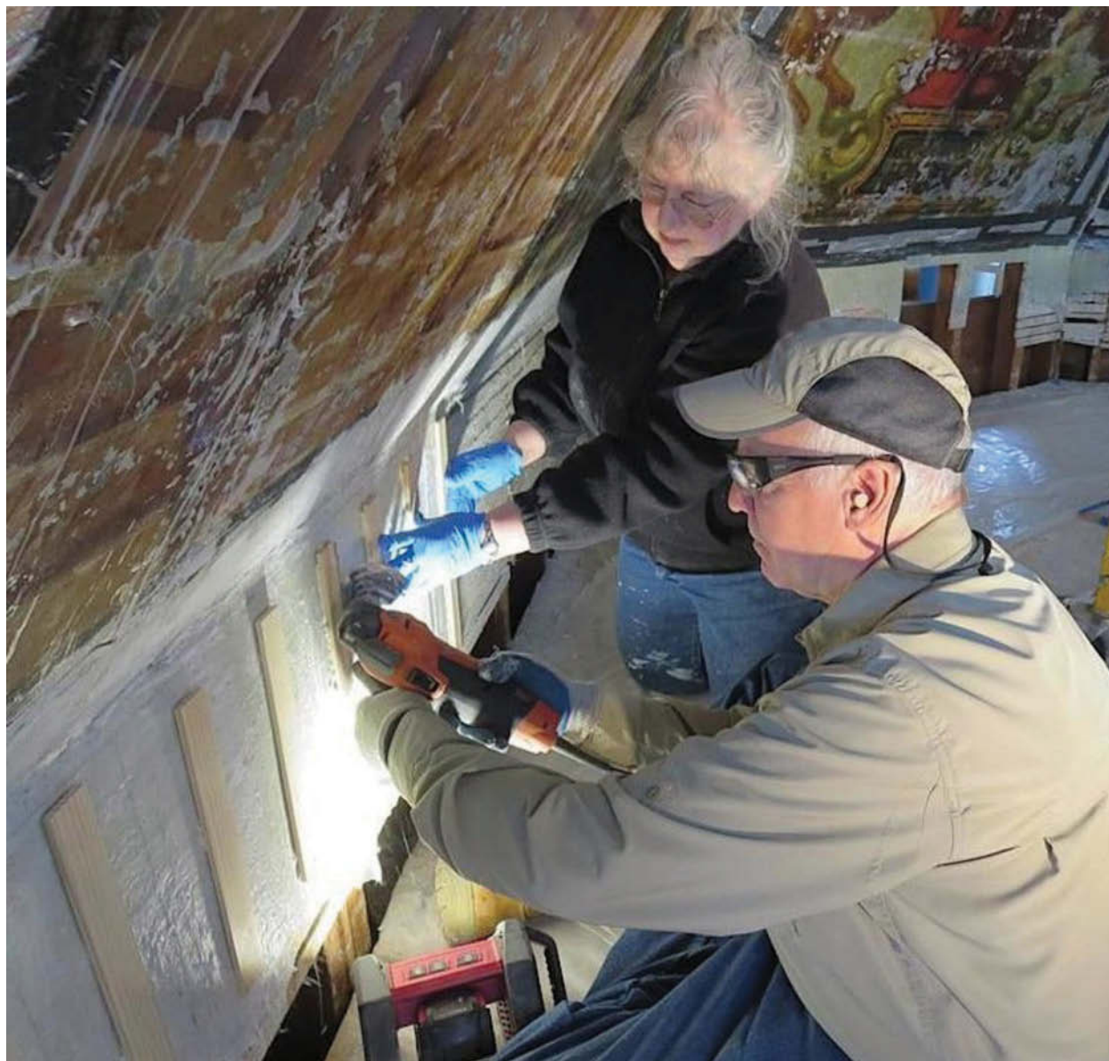
Fig. 12. Removal of painted plaster borders from lath (Courtesy of Lost Shul Mural Project)
