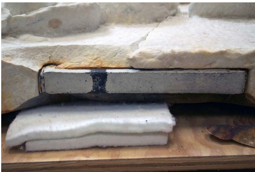
Fig. 6. The top cramp viewed from above showing its position slightly proud of the surface and the 3-mm gap in the stone around it (Photograph by Rachel C. Sabino, courtesy of the Art Institute of Chicago)
