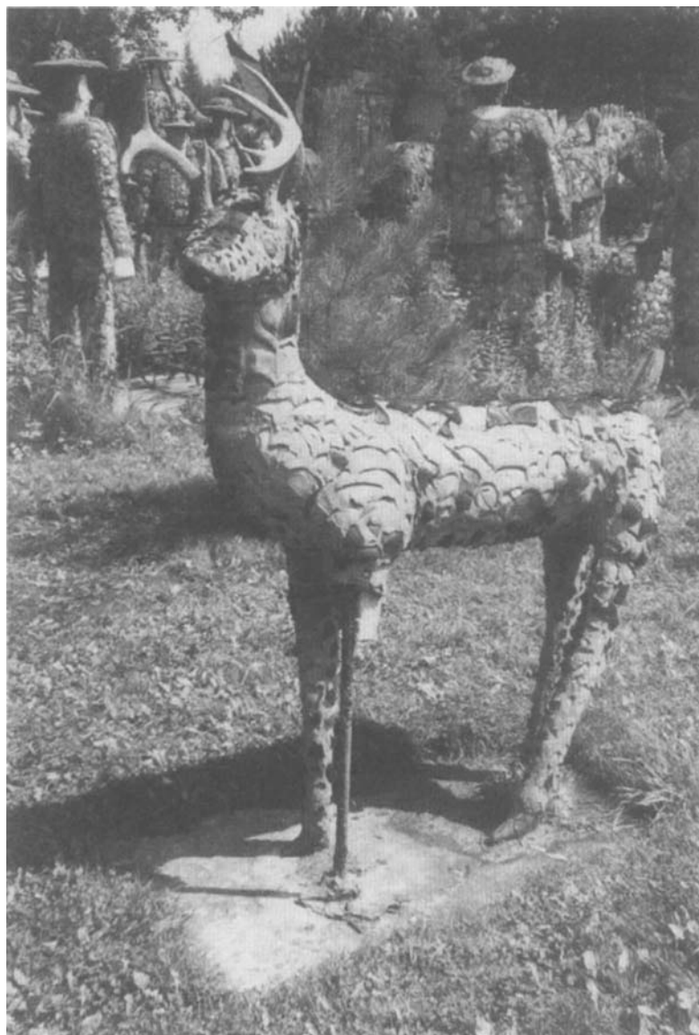
Figure 4. Wisconsin Concrete Park. Corroding iron armature has led to the deterioration of the concrete veneer.
