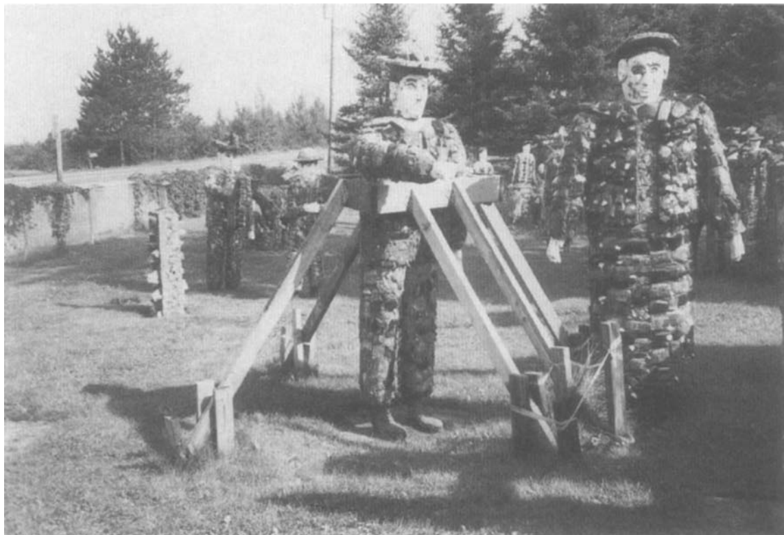
Figure 3. Wisconsin Concrete Park. Wooden braces support a weakening sculpture.
