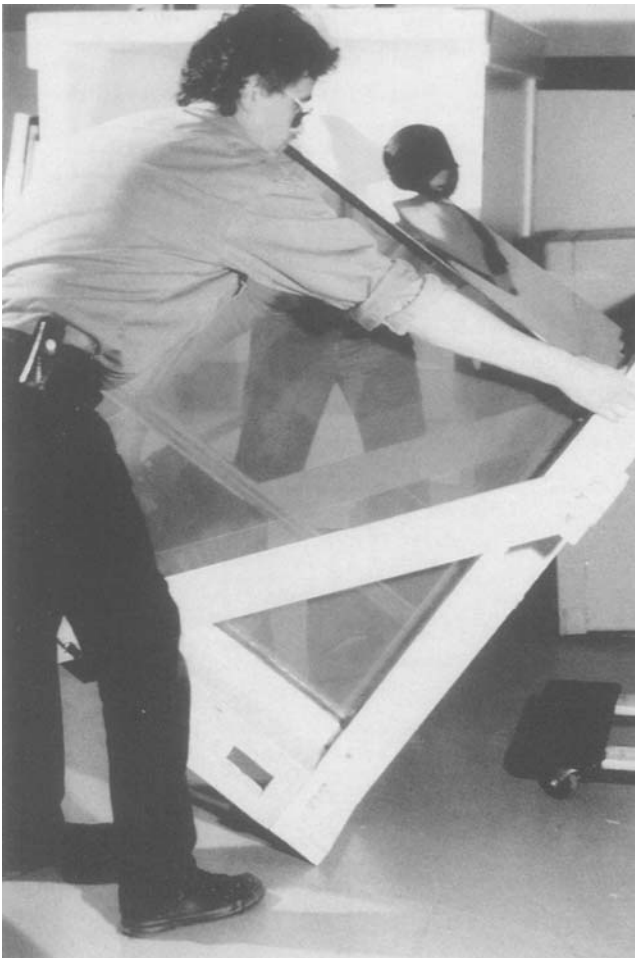
Figure 23. The two trays bolted and reinforced with cross bars are being rotated 90 degrees.
