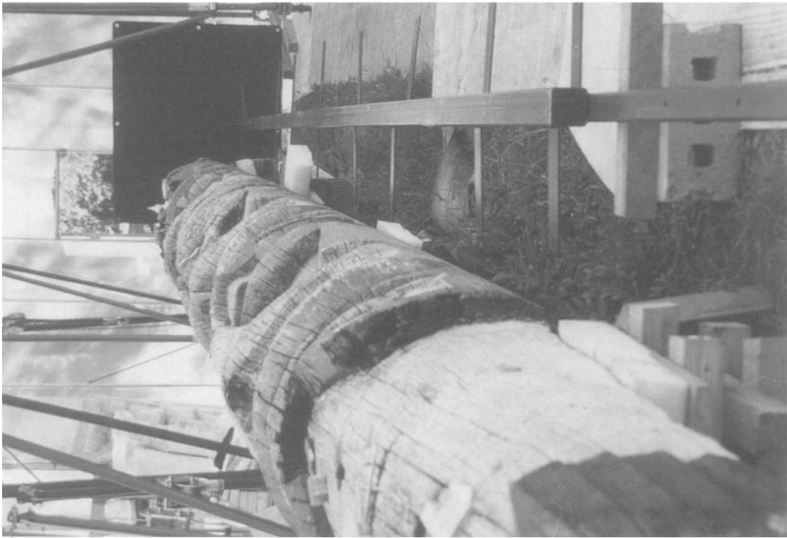
Figure 4. The pole and the strongback, prior to attachment.
