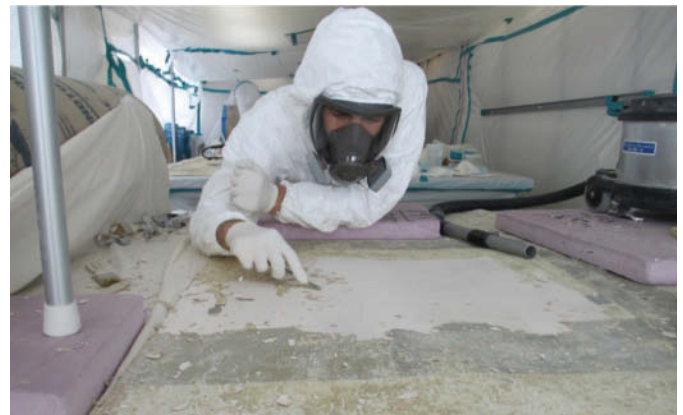
Figure 14. Manual overpaint removal
