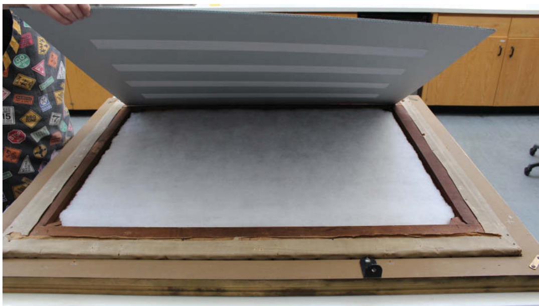
Figure 5. Option 1 for securing polyester batting to the backing board: backing board with attached Velcro strips is lowered onto reverse of the painting
