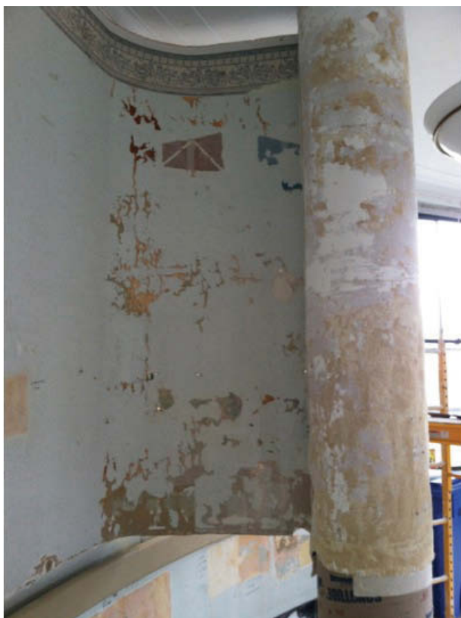
Figure 1. Mural on Sonotube being removed from wall
