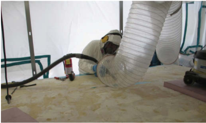
Figure 11. Lead adhesive removal with oscillating tool
