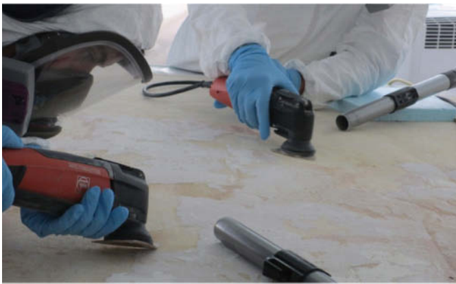
Figure 13. Lead adhesive removal with oscillating tool
