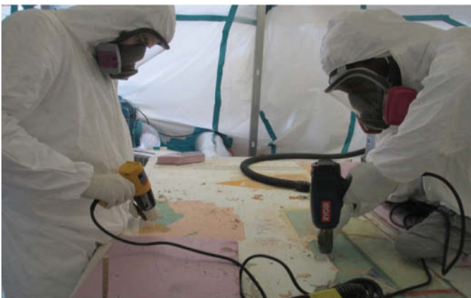
Figure 17. Overpaint removal
