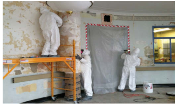
Figure 4. Mural removal in lead containment
