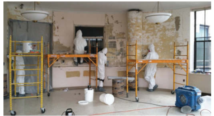
Figure 5. Mural removal in containment
