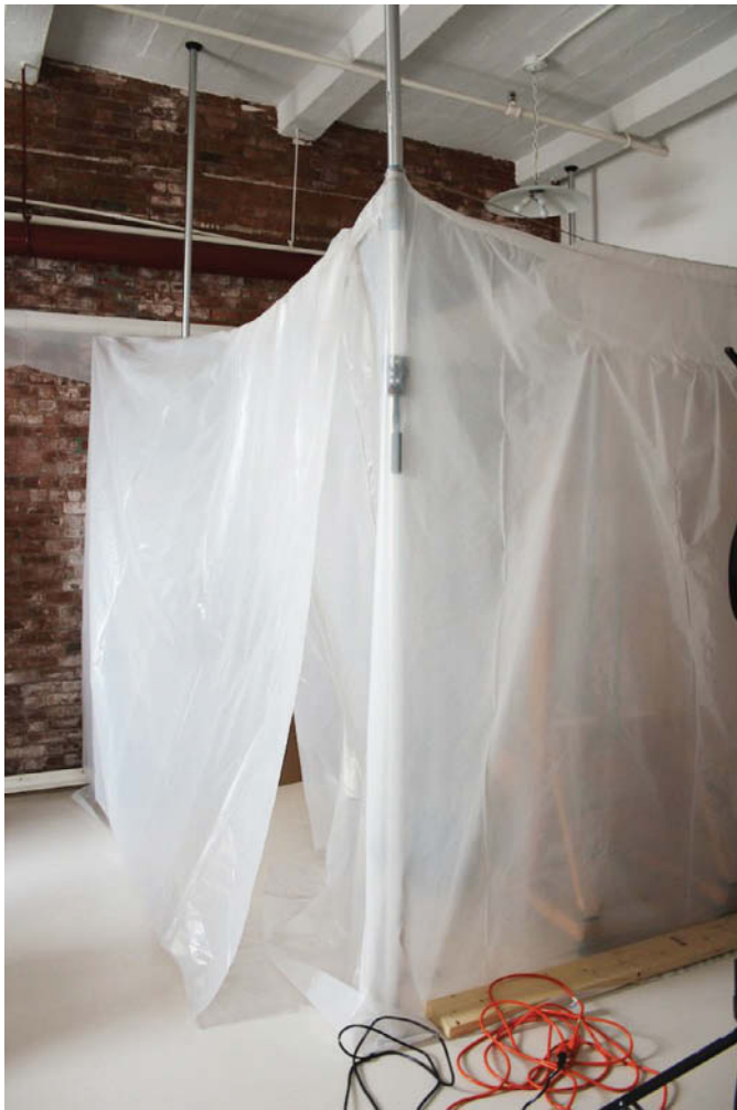
Figure 2. Temporary spray booth built in the studio with adjustable poles, plastic sheeting “walls” and paper protecting the floor
