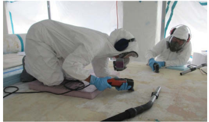
Figure 12. Lead adhesive removal with oscillating tool
