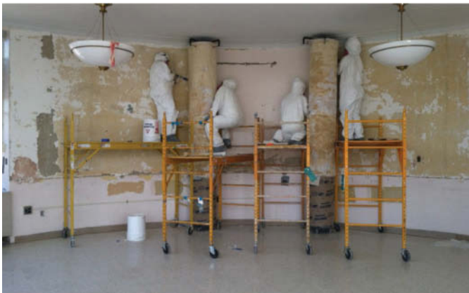
Figure 6. Final pieces of mural being removed in containment
