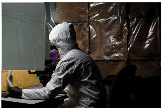
Figure 10. Inside lead containment space, with rare earth magnets securing polyethylene sheeting (inset).
