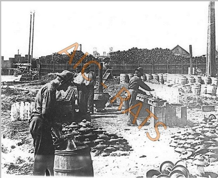
**Fabrication of Electrical Insulators Sealed with Sulfur**
