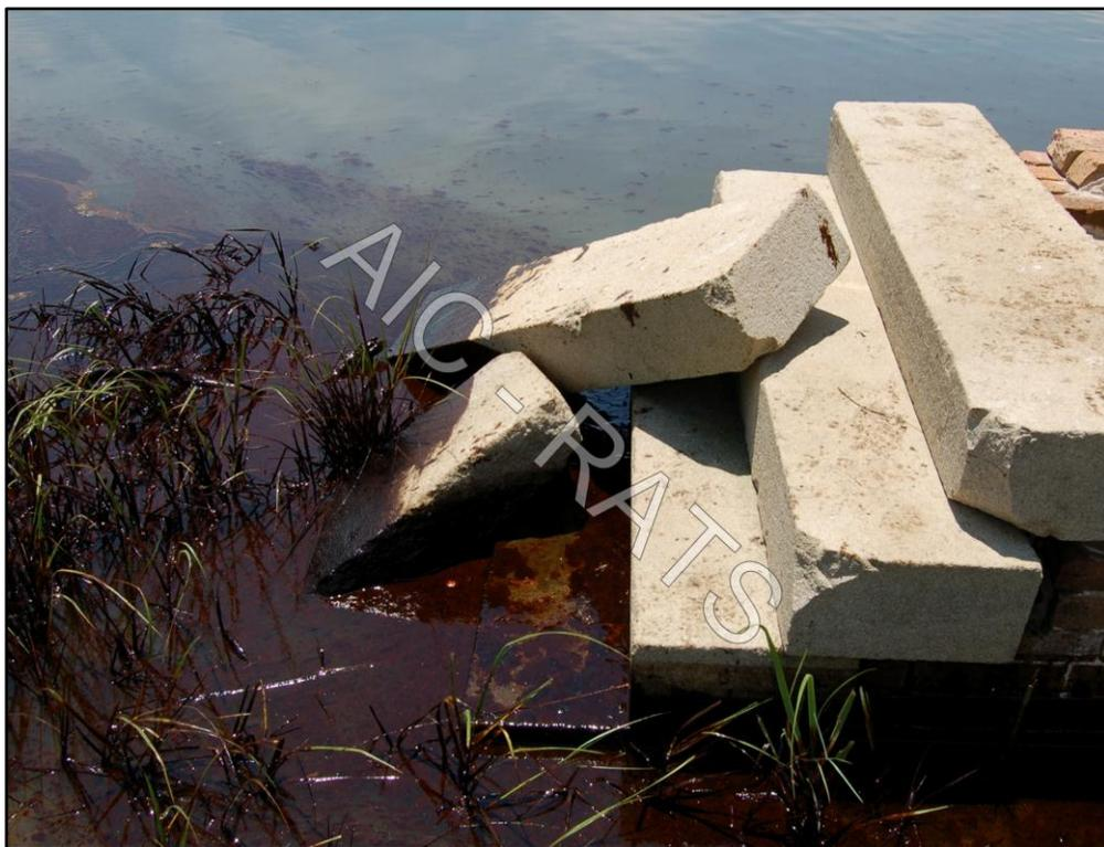
Crude oil on the granite stair treads and on the surface of the water. This is in the south facing bay that now adjoins the courtyard of the fort. The stairs lead up to the terreplein, the top surface of the ramparts on which cannon would have been placed. Note the contamination of the stair treads from oil transferred from boots/shoes.
