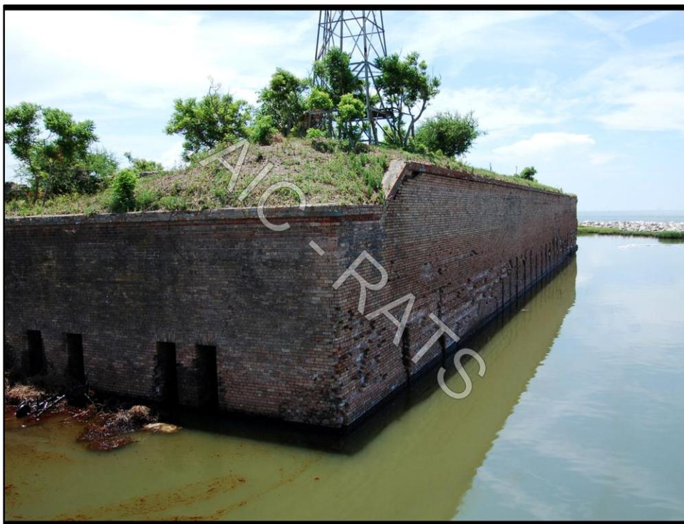
Northwest (left) and southwest (right) facing walls of the fort. The site is now protected by a rip-rap (mixed rock rubble) wavebreak visible in the background to the right. Note the oil sheen and globules on the surface of the water, and the debris that has collected against the wall to the left.
