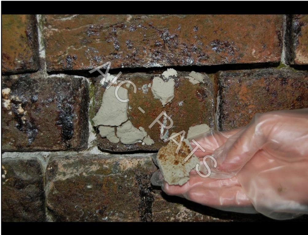
The clay poultice had dried slowly overnight. The cracked surface indicated that it was dry enough to remove. The piece that is being held shows some of the oil residue that was removed with the poultice.
