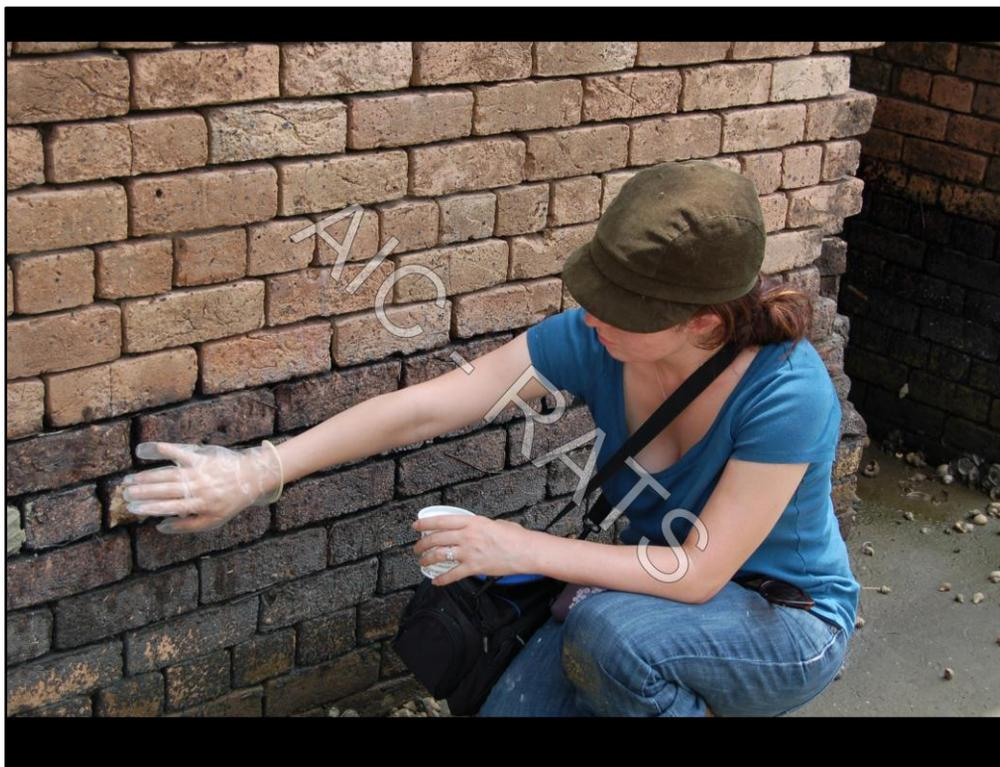
Erin White applying a poultice. A poultice method was also tested. A cleaner was mixed with a clay poultice to the consistency of peanut butter, applied, and allowed to dwell on the surface for approximately 16 hours. Once dry and beginning to crack, the poultice was flaked off and the surface was rinsed with clean water.
