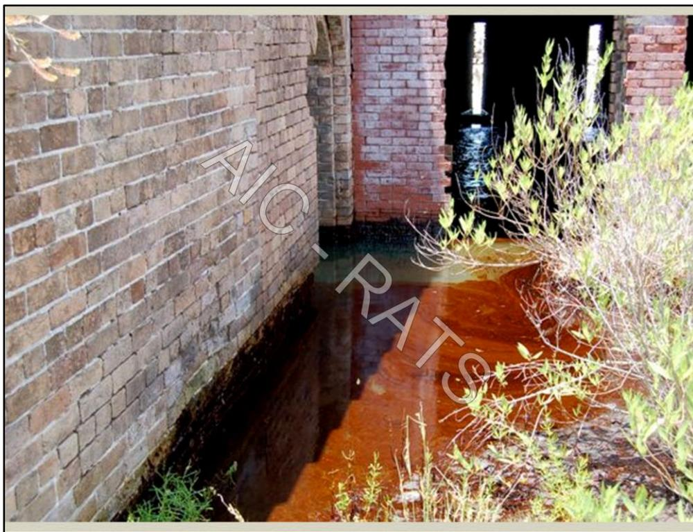
Looking southwest inside the fort, water intrudes into the fort during high tide. In the foreground is the corner of the interior courtyard. In the background is one of the casemates (fortified gun emplacements) that has been contaminated with oil.
