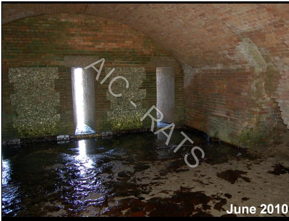
Looking west in the same room, June 2010, showing patches of oil stranded on the sand that has been deposited over the floor of this room over time.
