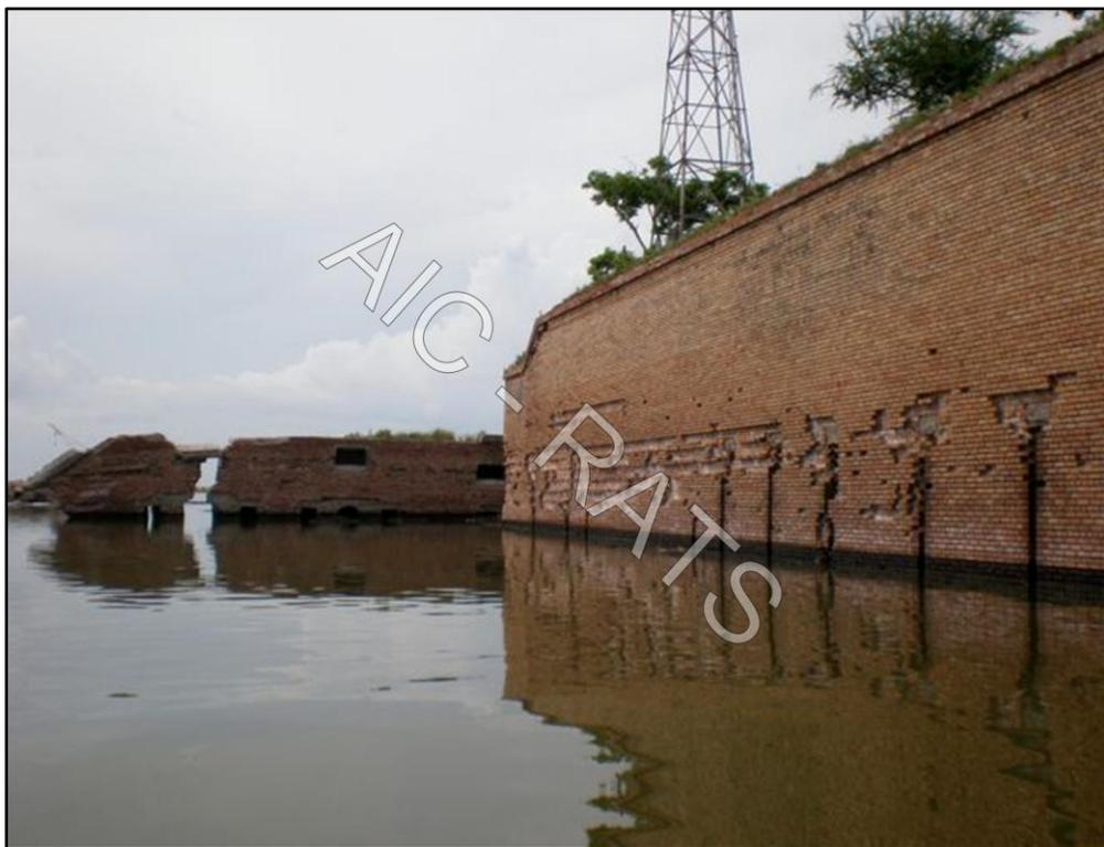
Southwest facing wall showing the condition of the exterior brick walls and the oily “bathtub ring” at the base.
