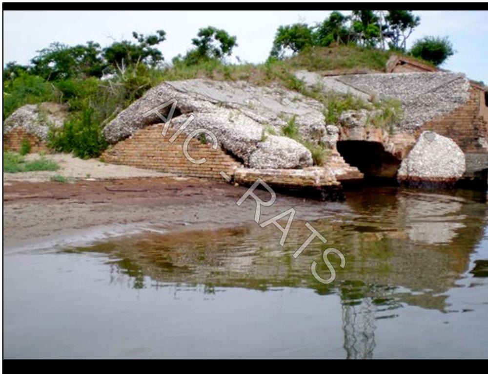
Storm damage has exposed the tabby walls (tabby is a unique Southern coastal building material made from a mixture of lime, sand, and oyster shells ). A bathtub ring of oil can be seen on the southern, partially submerged portions of the fort, and is obvious at the high water line on the beach to the left in the photo.
