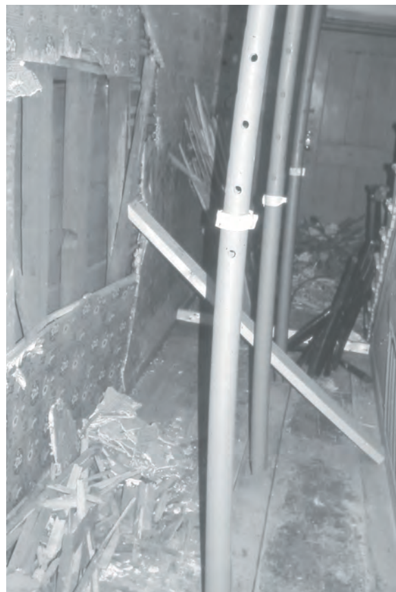
Figure 2. Structural engineers propped up the sagging structure.
