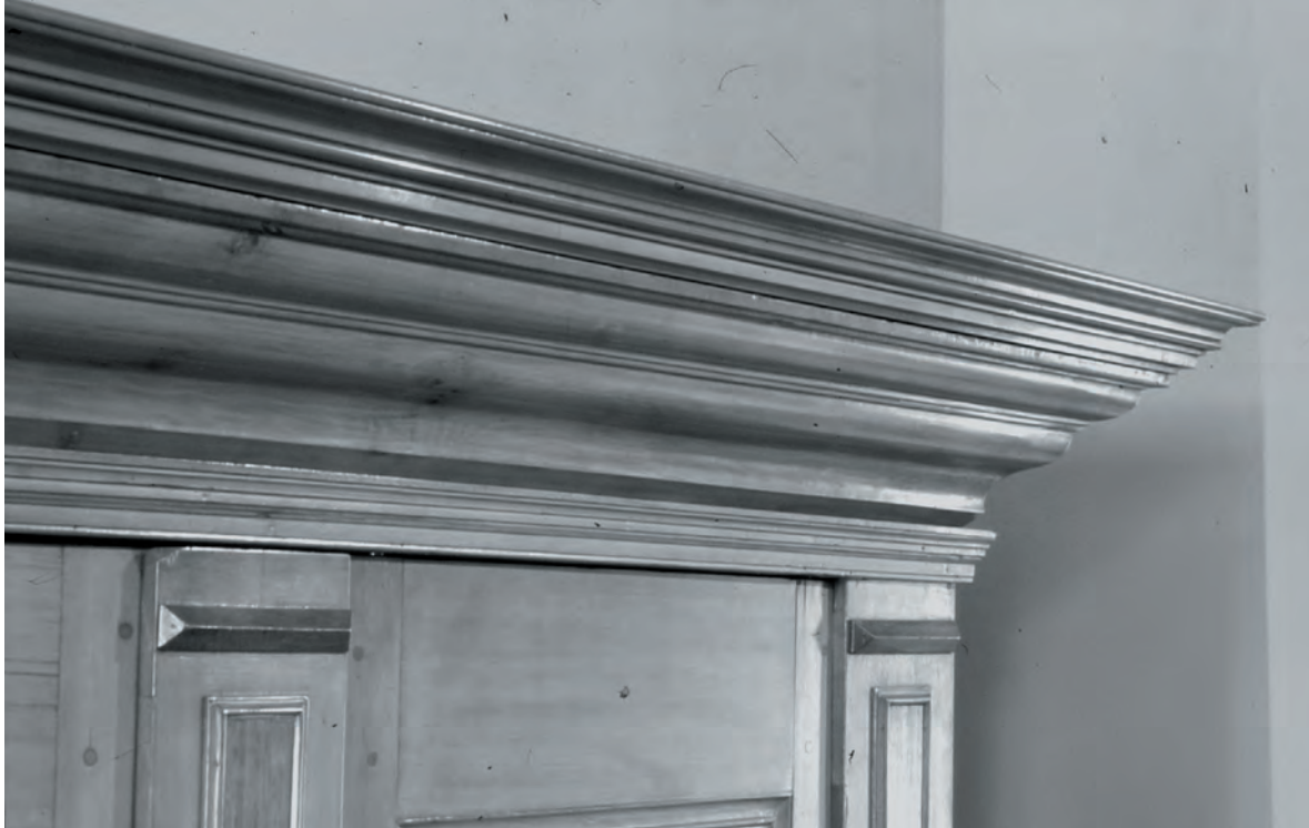
Figure 10. The cornice with the removable restoration completed.
