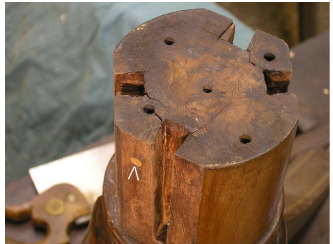
Fig. 7. Bottom of the pedestal column showing cracks where the stress on the legs split the wood. The 5 holes are from the screws holding a reinforcing metal plate. The white circle (arrow) is the end of a dowel from a previous repair to strengthen the column.
