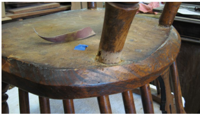
Fig. 20. The leg glued in place. A ring of finish has been sanded off in preparation for the band of carbon fiber-reinforced epoxy.
