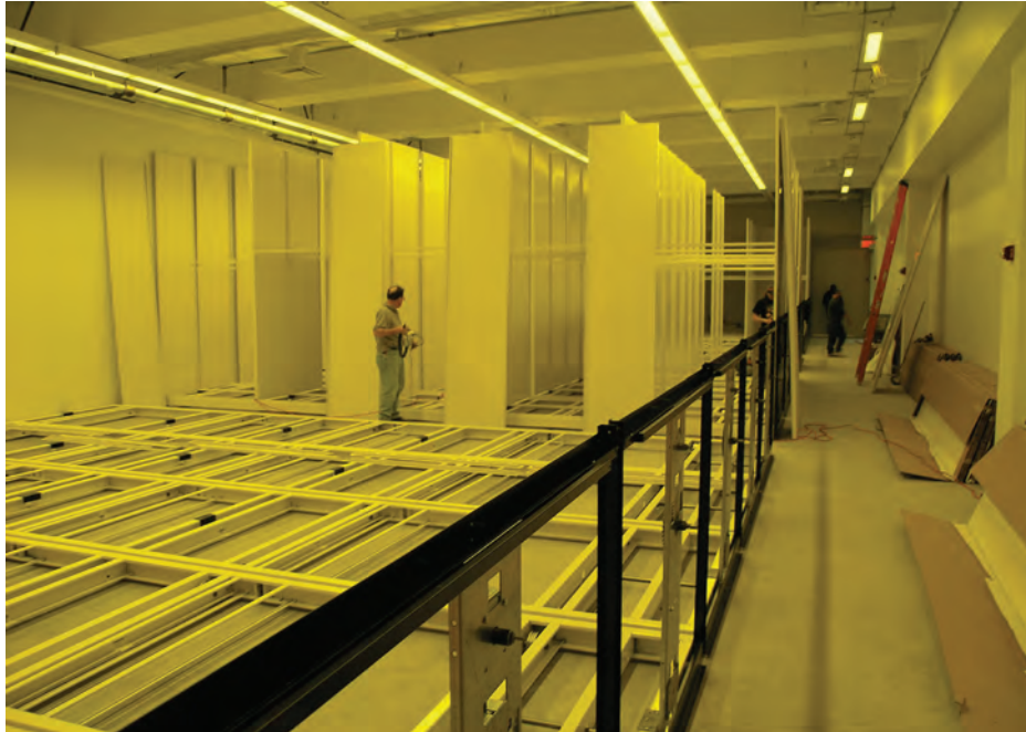
Figure 11. Shelving skeletons prior to installation of sides and backs.
