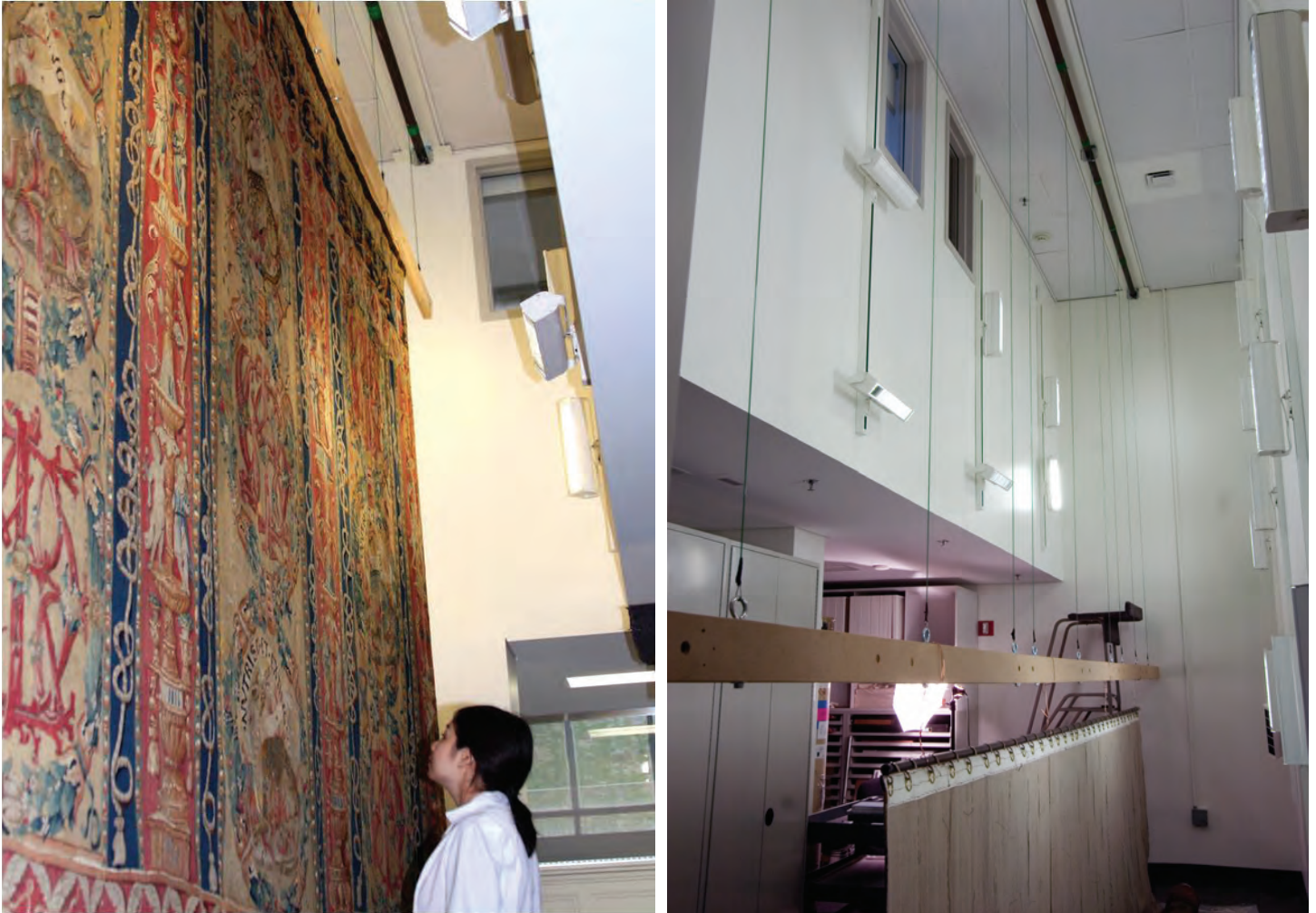
Figure 5. High Ceiling work space has electronic hoist for examination and treatment of large textiles (hoist lowered at right). Lighting is provided by adjustable light fixtures on vertical tracks.
