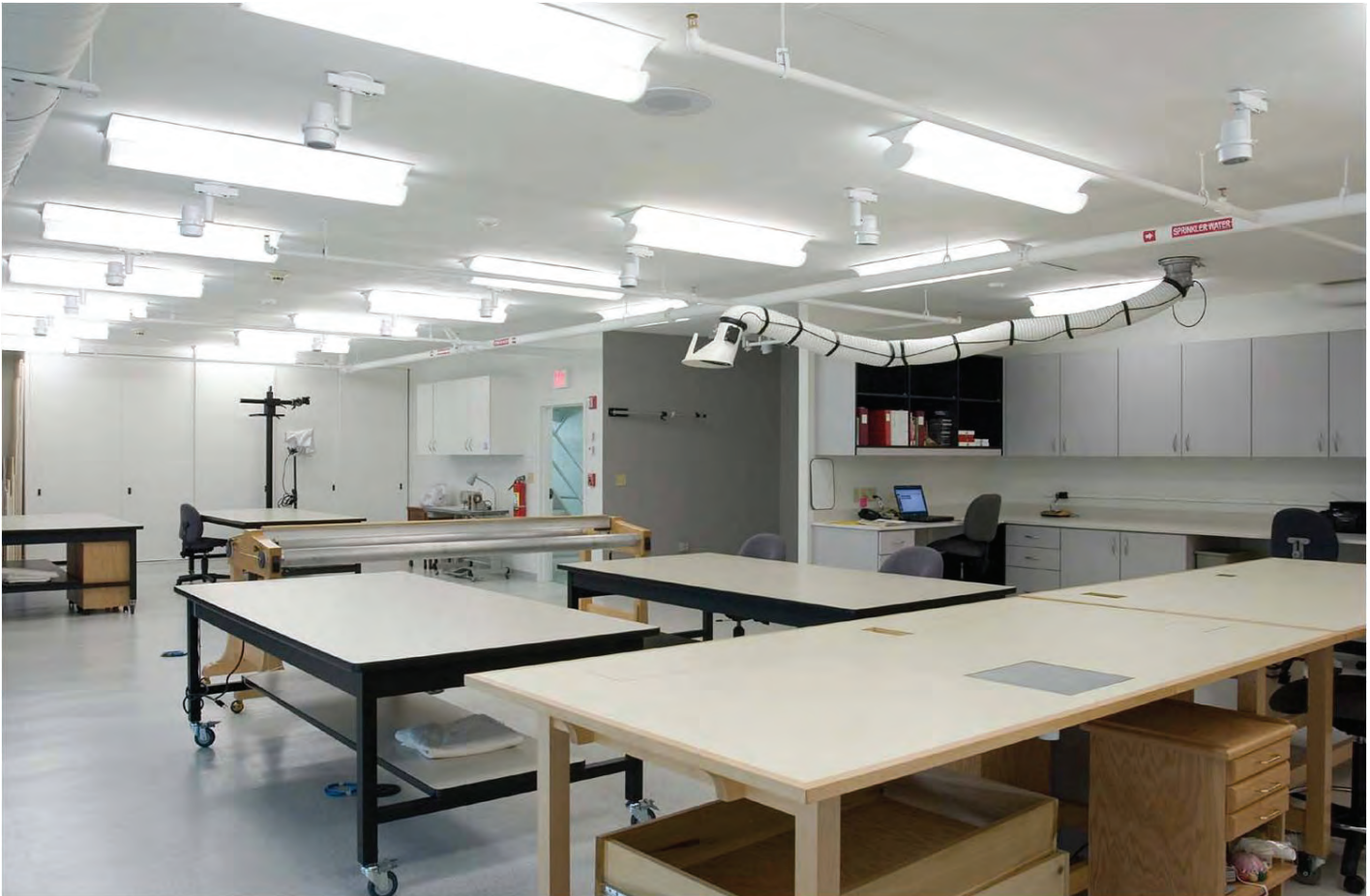
Figure 3. Dry conservation area with ceiling mounted Nederman exhaust trunk, and two types of tables.
