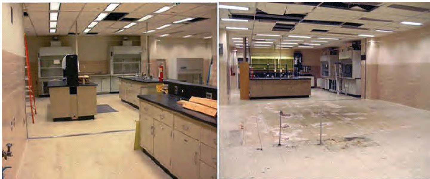
Figure 2. G52 Laboratory Re-Construction.
